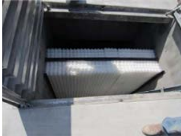
Typical Coalescing Separator
