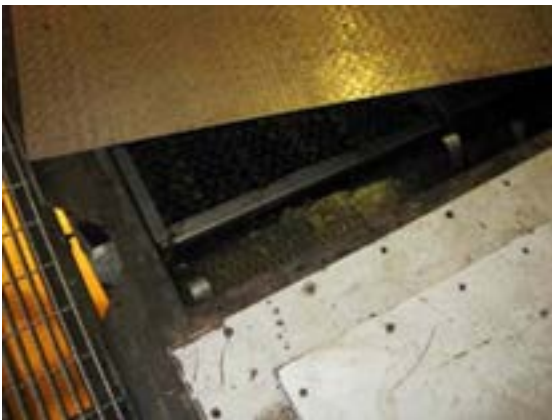
Separator with Old Media and Little Oil Collected on top of Water
