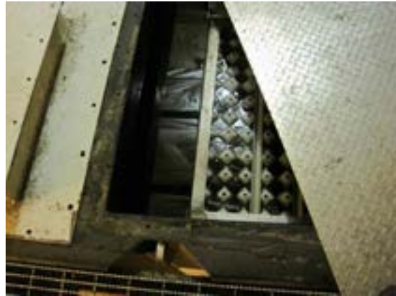
Separator with new media and large quantities of collected oil
