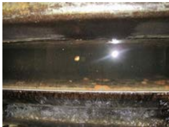
New media separator water overflow with little or no bacterial growth
