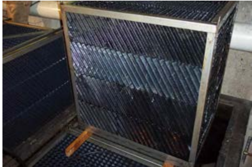
Logs of media installed in one of the frames
