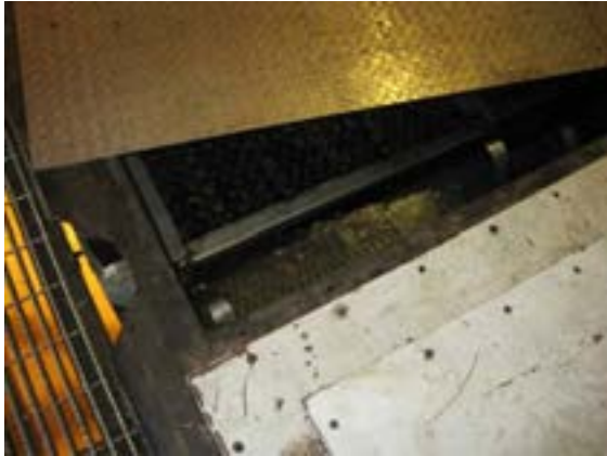
Separator with old media and little collected oil on top of water
