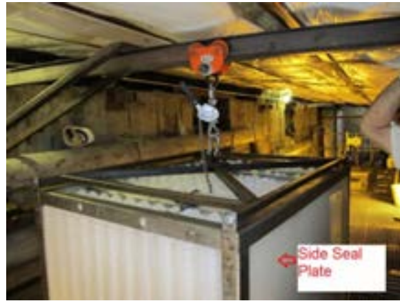
Lowering Pack into Separator
