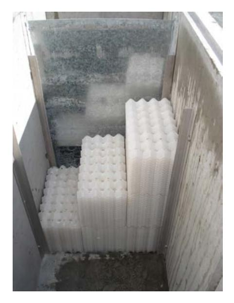
Coalescing Modules are installed against one wall of vault
