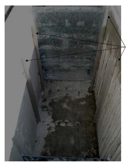
Stainless steel or fiberglass material side rails are installed to side walls fore and aft of the coalescing plate area, approximately 24 inches (625 mm) apart, a little ahead of the oil dam
