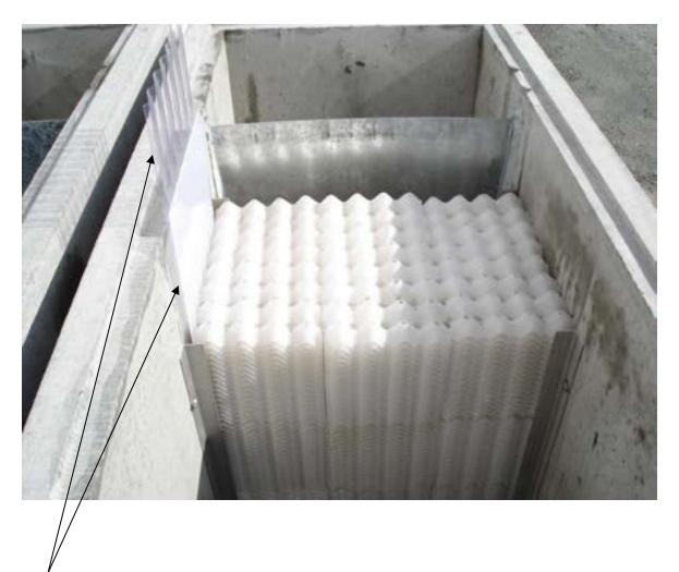
Side Sealing is accomplished with flat plate and wavy spring plate to ensure flow must pass through the coalescing media.
