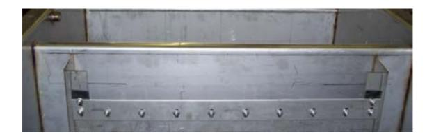
Adjust overflow weir by loosening bolts, sliding to desired elevation and retightening bolts. Be sure weir is level.
