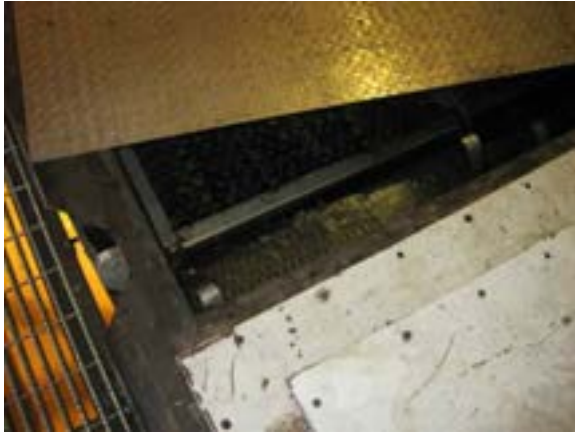
Separator with Old Media and Little Oil Collected on Top of Water
