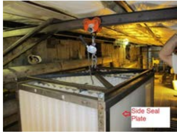
Lowering Pack into Separator
