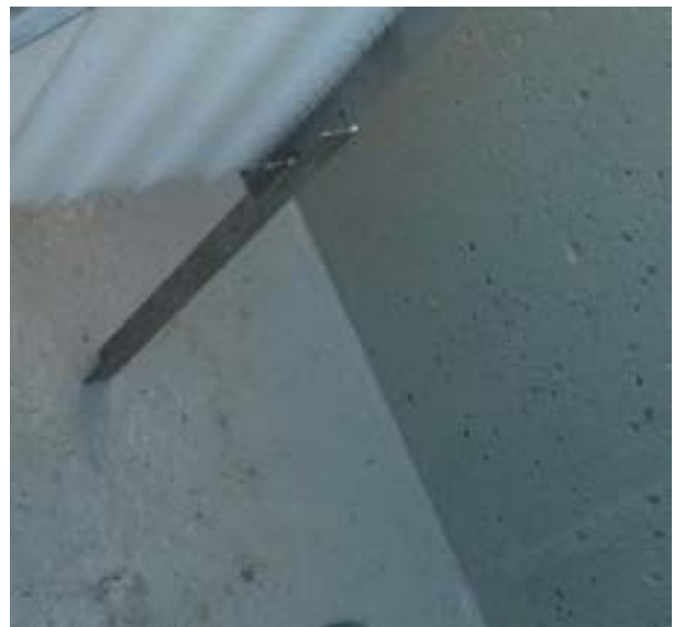
Outlet end of Insert with support leg showing outlet solids accumulation area
