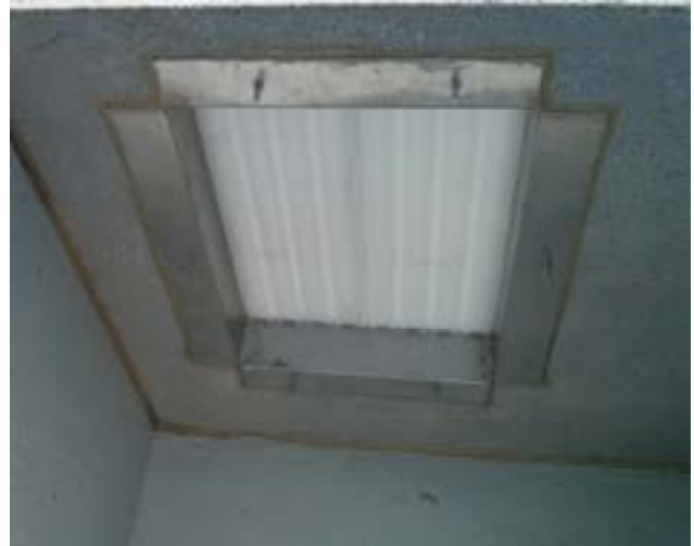
Inlet end of Insert with sealant and showing inlet solids accumulation area
