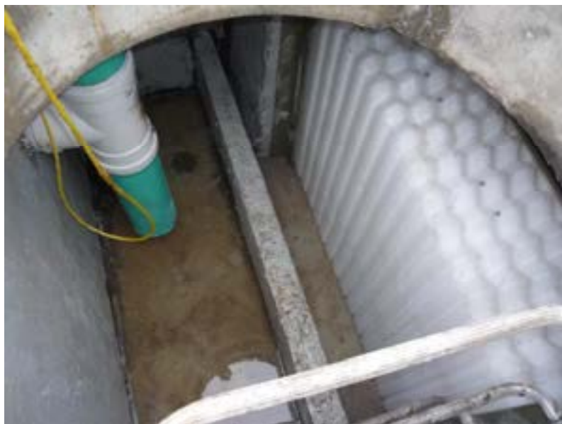
Hydro Transformer Storage facility
