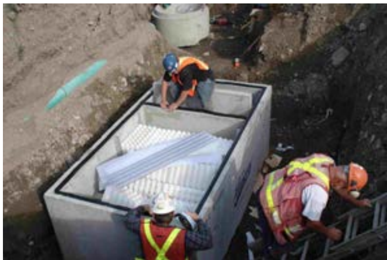
Hydro Storage Facility
