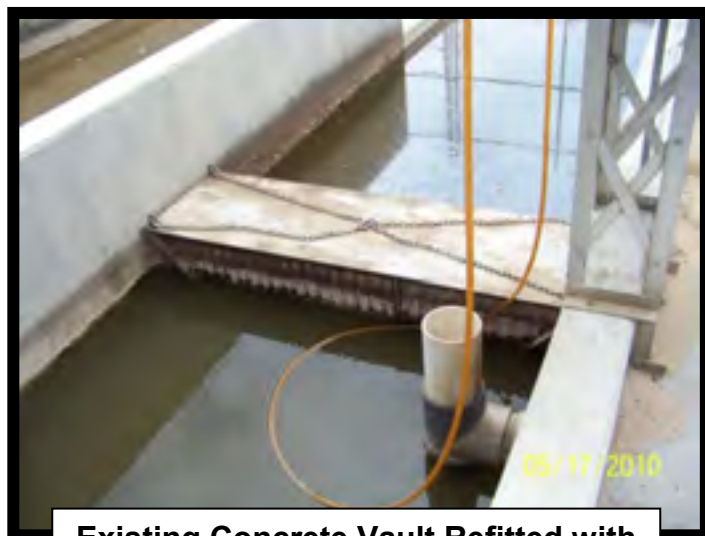
Existing Concrete Vault Refitted with Coalescing Media Frame System
