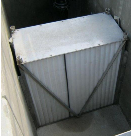
Typical Below-Ground Installation Frame Type of Coalescing Media System
