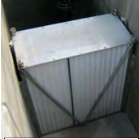
Typical Below-Ground Installation Frame Type of Coalescing Media System
