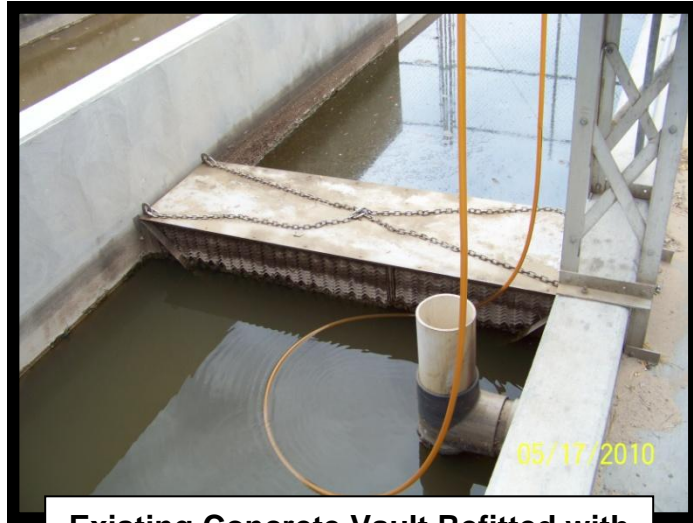
Existing Concrete Vault Refitted with Coalescing Media Frame System
