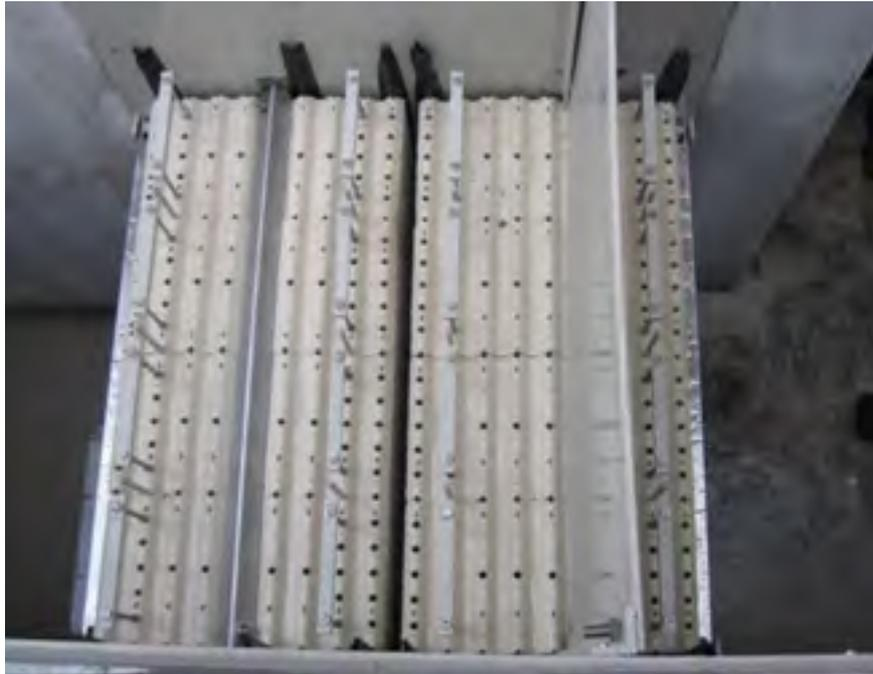
Figure 5: Typical Horizontal Corrugated Plate Installation
