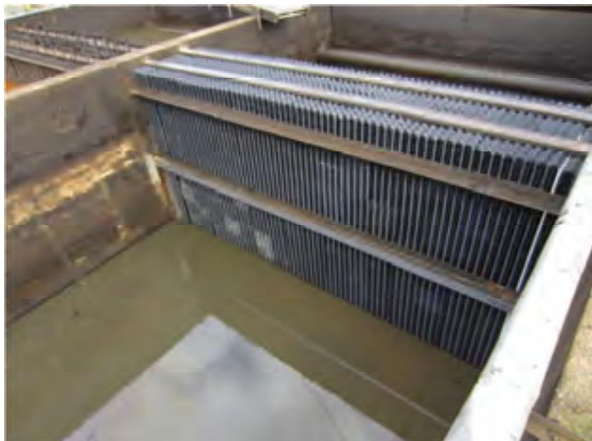
Figure 8 API Retrofit in Refinery
