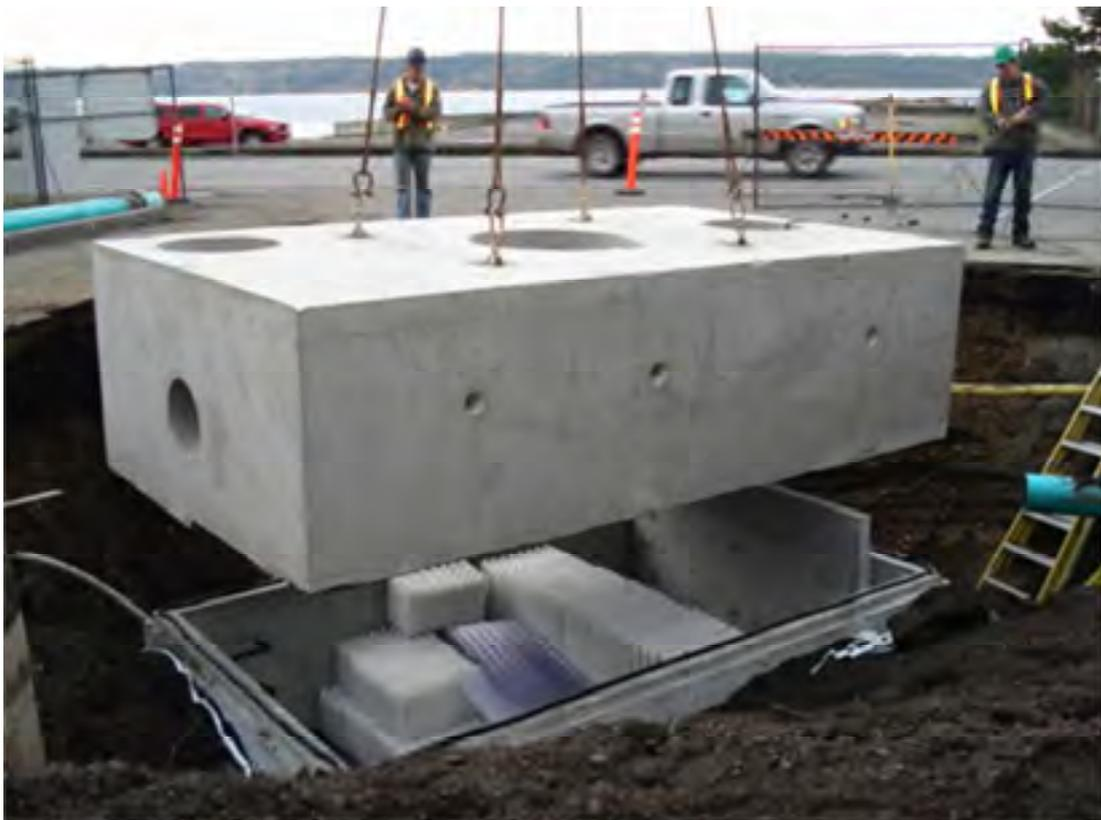
Figure 7: Typical Vault Utilizing Multiple Angle Plates, Partially Assembled
