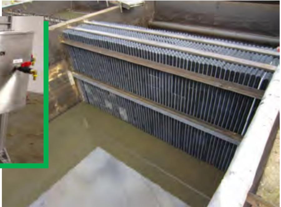
Oil Refinery Effluent Separator: One of a set of four—total capacity 20,000 US gpm (4600 m<sup>3</sup>/hr)
