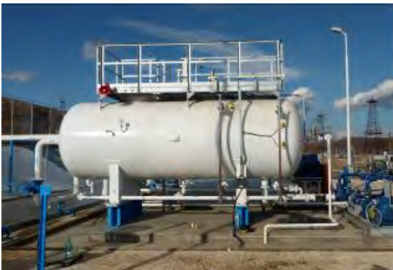
MSR DESIGN OIL PRODUCTION SEPARATOR (ROMANIA)
